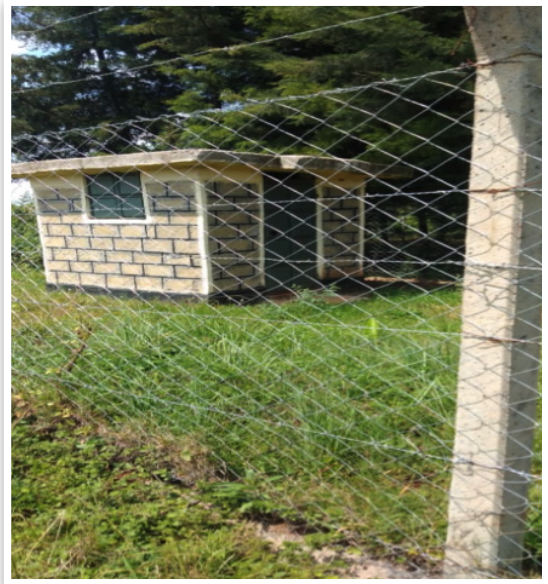
Figure 16: Chepkemel Water Project power House
