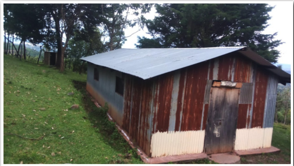
Figure 2: One of the Dormitory Structures at Toroton VTC
