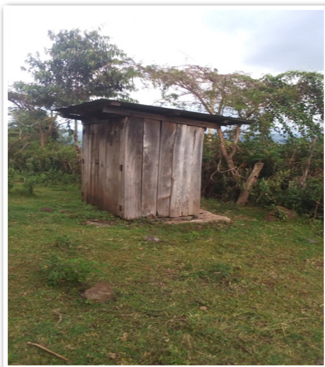
Figure 4: A latrine used by Trainees Boarding at Toroton VTC
