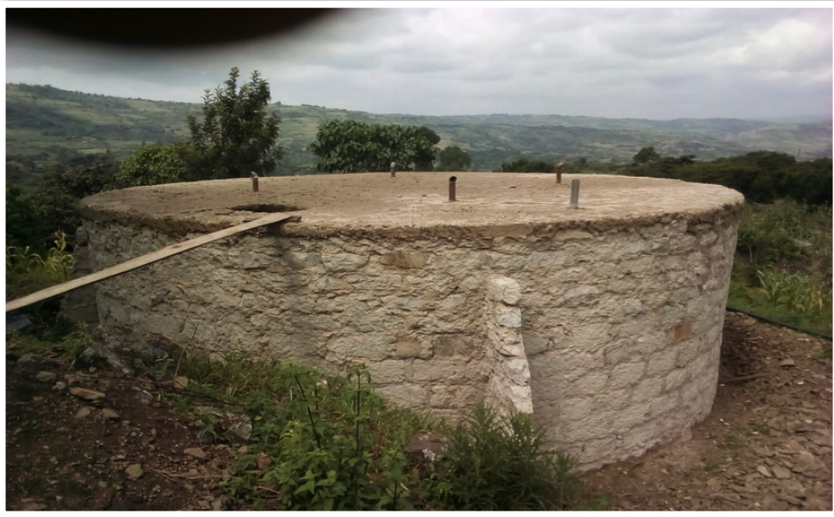
Figure 12: The Water Tank for Kapkures Water Project
