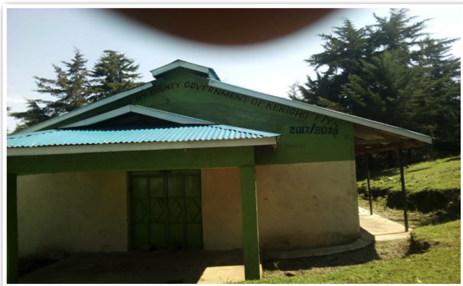
Figure 1: A newly built workshop at Toroton Vocational Training Centre
