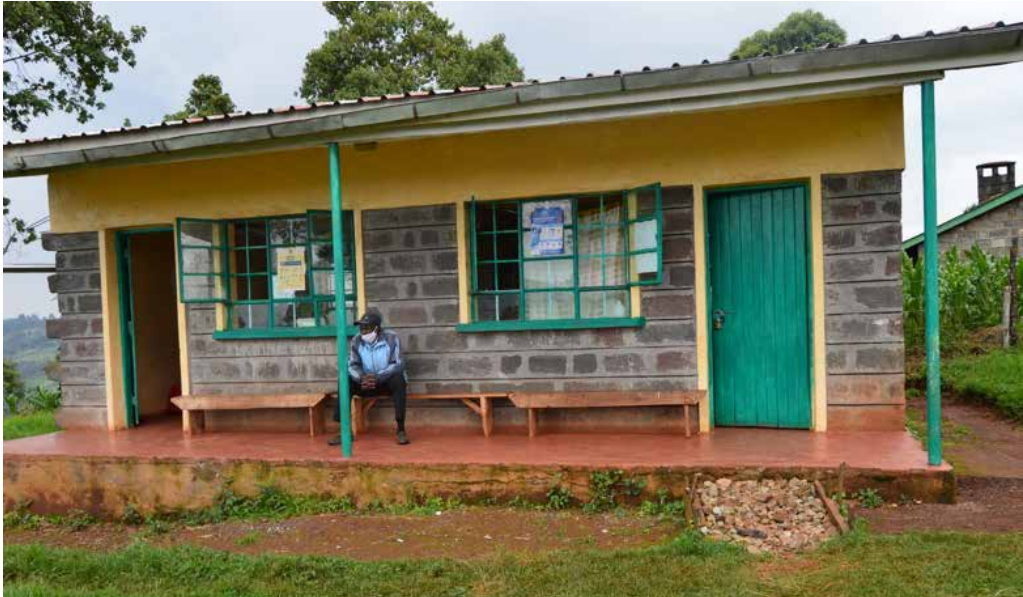
Figure 7: Main building – consultation room and treatment room- at Ndoinet Dispensary
