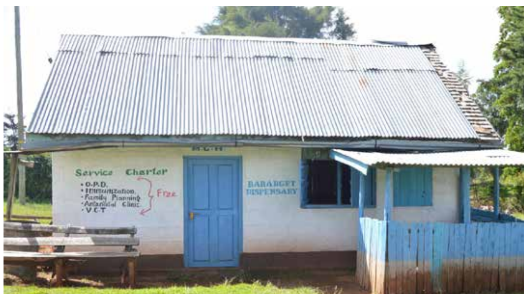
Figure 1: Service rooms at Bararget Dispensary
